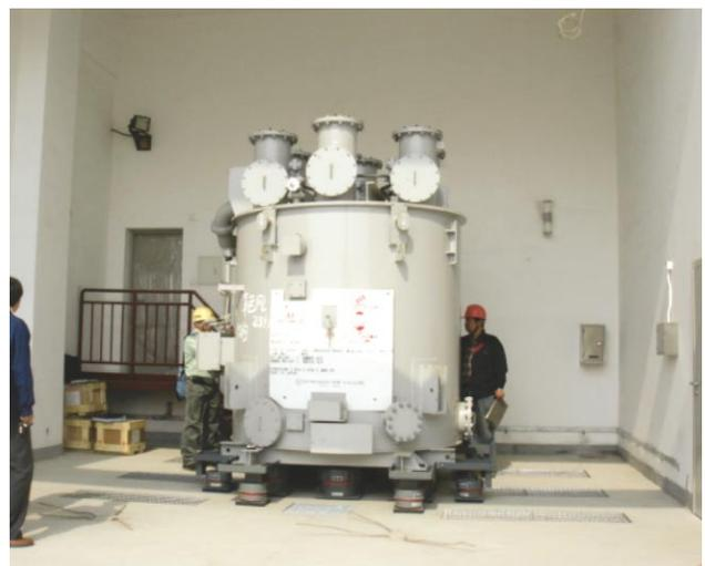
図3 ShR 37kV 20MVar (組立て中)
