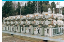
154kV Gas Insulated Switchgear
