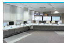
Supervisory Control System for Expressways
