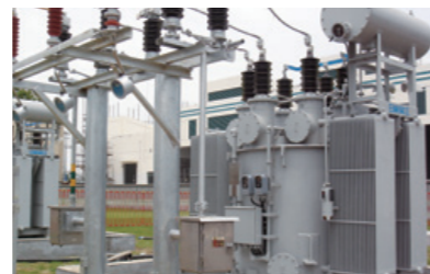
Shunt Reactor
