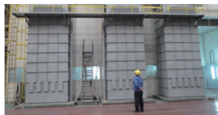
Installation of fume purification system inside painting facility
